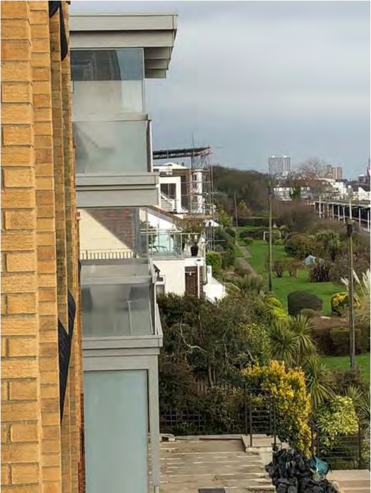
Photo of both south balconies showing clear glass on 31/3/18
